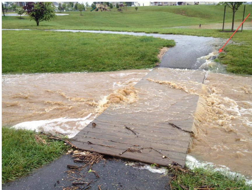
FIGURE 6: Across from the bridge, water can be seen running down the walking path.
