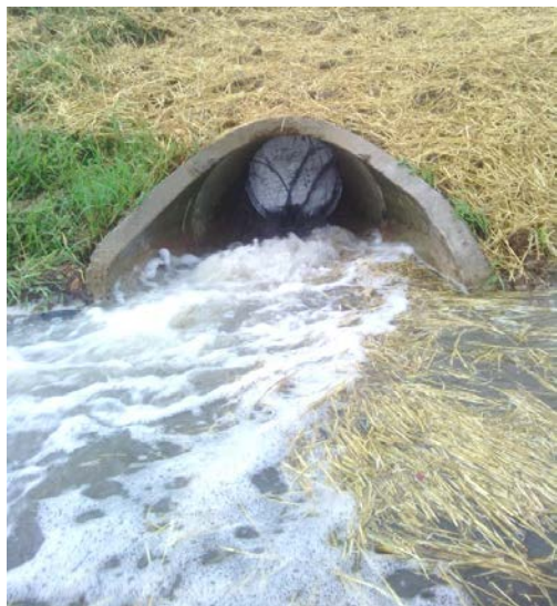
FIGURE 3: The lightly shaded area seen inside the pipe is an orifice plate to limit stormwater flow to the forebay. Limiting flow to the forebay directs more water to the lake.
