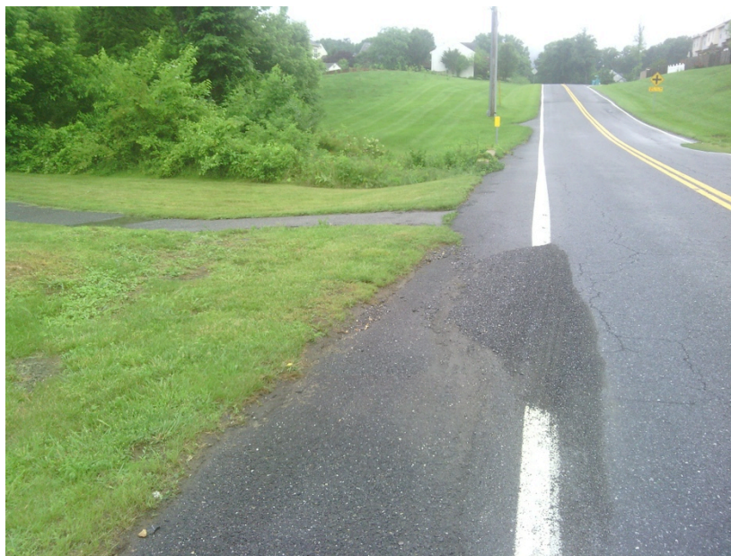
FIGURE 10: Runoff from the road needs to be directed to the stream. Developer work on the nearby culvert may solve this problem.
