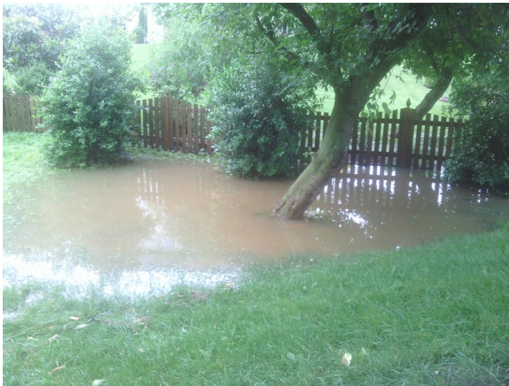
FIGURE 9: Flooded back yard on Canal Clipper Court due runoff from Ballenger Creek Pike.
