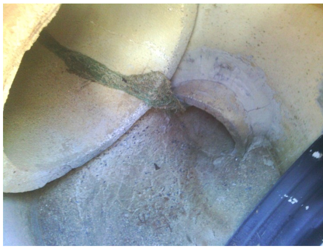
FIGURE 5: Due to its contoured shape, the splitter near the clubhouse will be more difficult to restrict as was done in Figure 4. The HOA should seek out cost estimates.
