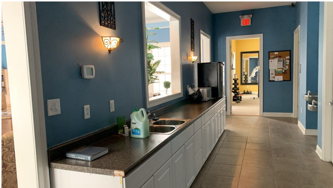
Building Interior - Kitchen, Remodel
